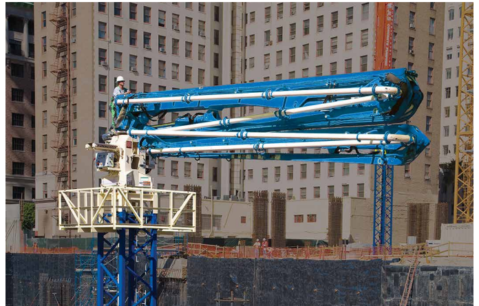
STEP 4 – Position, pin and pump
