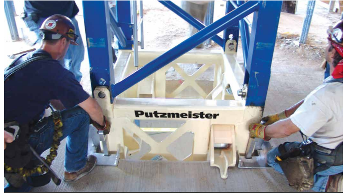
SIMPLE BRACING WITH VERTICAL SUPPORT
